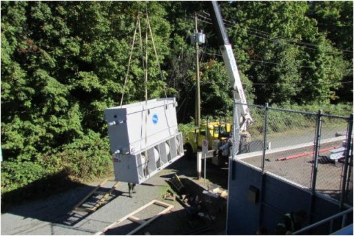
New condenser loading on to the roof, replaced two old condensers
