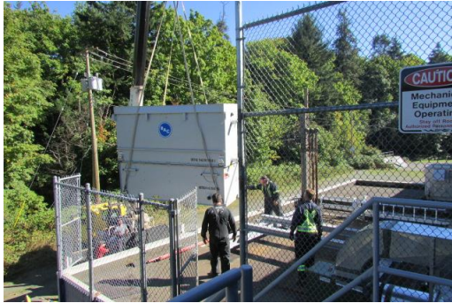
New condenser loading on to the roof, replaced two old condensers
